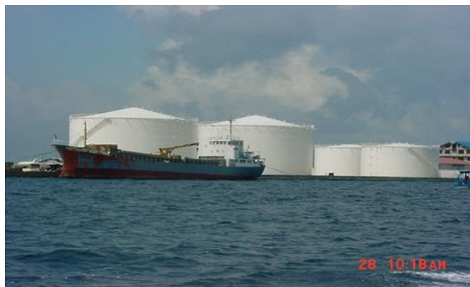
Petroleum Storage Tank Farms
