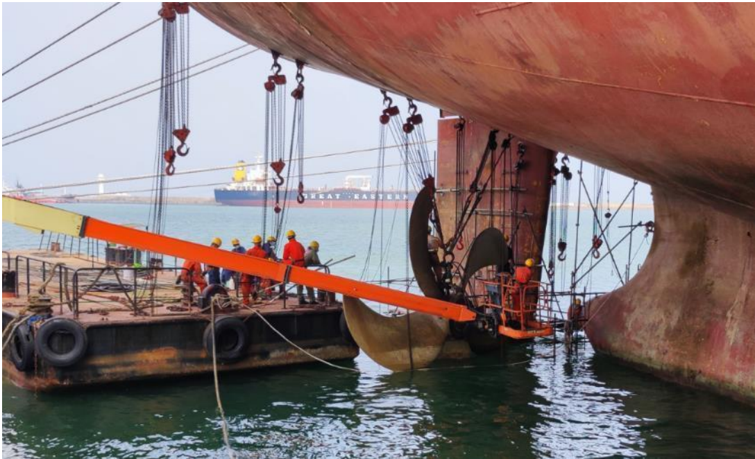
Unique repair solutions from RRARS – commencing docking repairs while afloat
