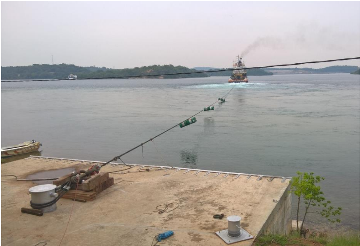
Trincomalee Bollard Pulling Facility
