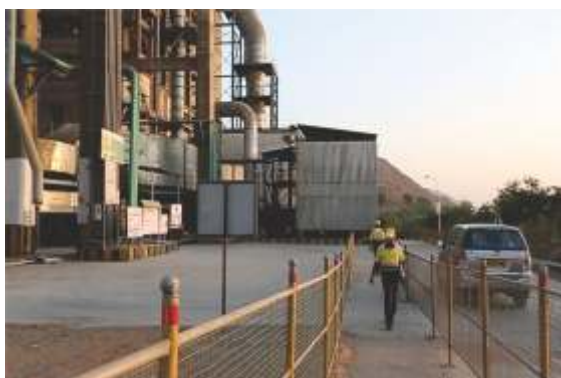
Good safety practice – designated pedestrian pathways inside the plant
