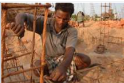
Habitat home partner at a construction site for his home
